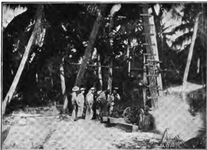
FIG. 26.—The Site of the First Boring, with Derrick and Machinery.
